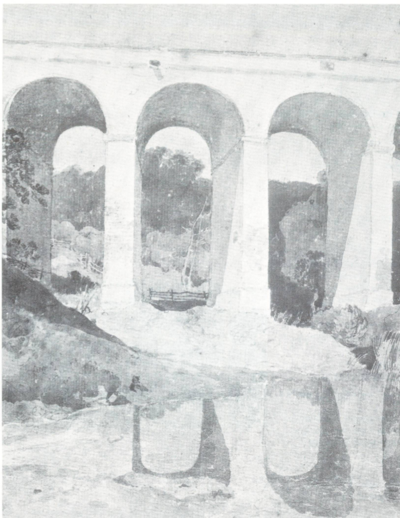
John Sell Cotman, Chirk Aqueduct , 1806–1807, The Board of Trustees of the Victoria and Albert Museum, London
