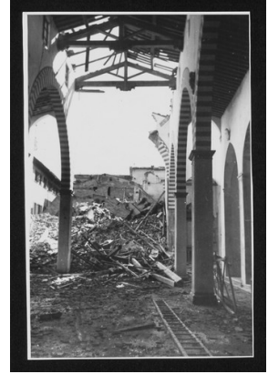
SC-016_13979_016.tif Damaged monuments E
