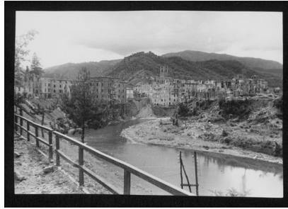
SC-016_13977_032.tif Damaged monuments C
