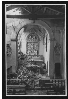
SC-016_13985_007.tif Damaged monuments P
