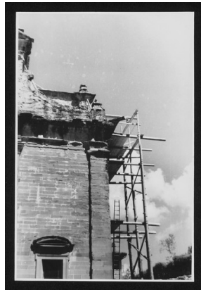
SC-016_13977_065.tif Damaged monuments C
