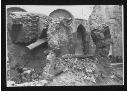
SC-016_13976_014.tif Damaged monuments B
