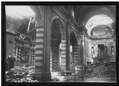
SC-016_13977_037.tif Damaged monuments C
