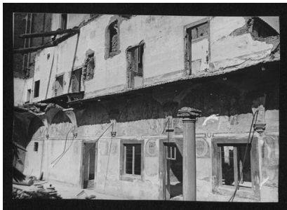
SC-016_13985_072.tif Damaged monuments P
