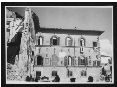
SC-016_13985_045.tif Damaged monuments P
