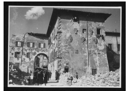
SC-016_13985_044.tif Damaged monuments P
