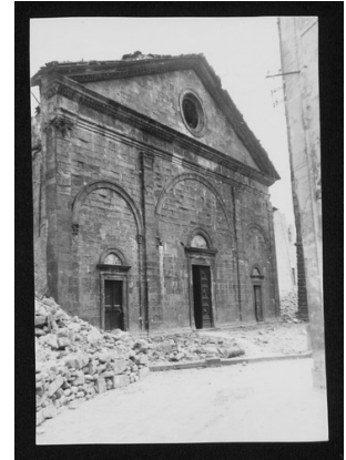
SC-016_13977_033.tif Damaged monuments C
