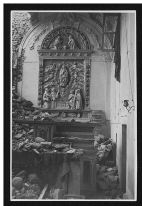
SC-016_13985_009.tif Damaged monuments P
