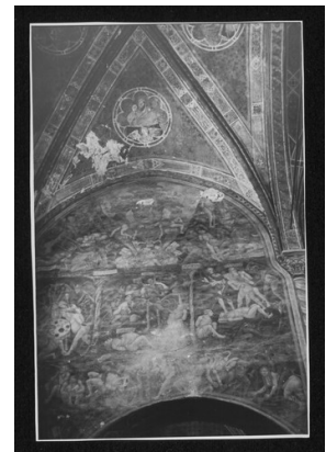
SC-016_13987_069.tif Damaged monuments S
