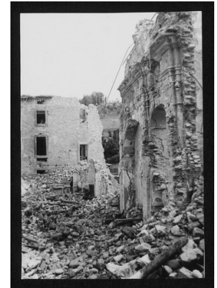
SC-016_13977_036.tif Damaged monuments C
