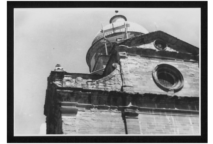
SC-016_13977_064.tif Damaged monuments C
