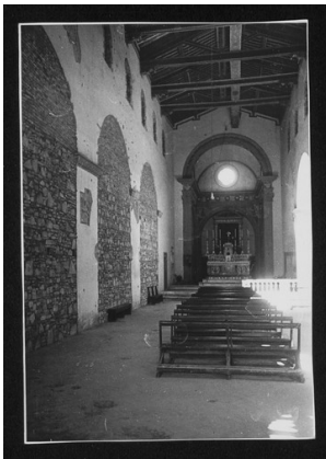
SC-016_13976_017.tif Damaged monuments B
