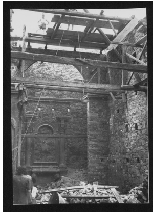
SC-016_13979_018.tif Damaged monuments E
