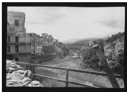
SC-016_13977_038.tif Damaged monuments C
