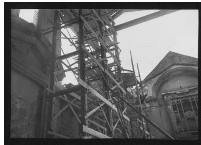
SC-016_13985_079.tif Damaged monuments P
