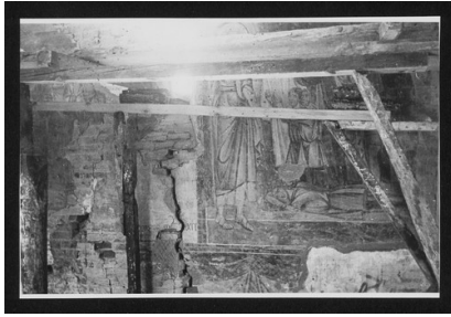
SC-016_13985_102.tif Damaged monuments P
