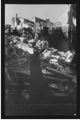
SC-016_13979_014.tif Damaged monuments E
