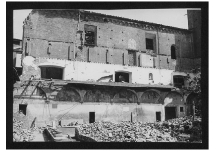
SC-016_13985_041.tif Damaged monuments P
