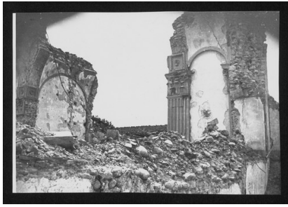
SC-016_13985_039.tif Damaged monuments P
