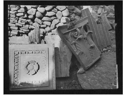
SC-016_13985_095.tif Damaged monuments P
