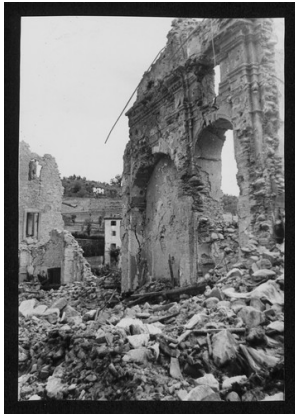
SC-016_13977_034.tif Damaged monuments C
