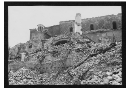
SC-016_13977_039.tif Damaged monuments C
