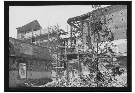
SC-016_13985_077.tif Damaged monuments P
