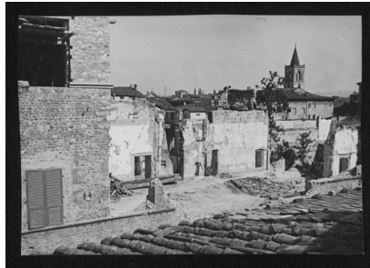
SC-016_13985_070.tif Damaged monuments P
