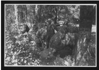
SC-016_13985_006.tif Damaged monuments P
