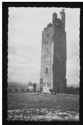
SC-016_13987_041.tif Damaged monuments S
