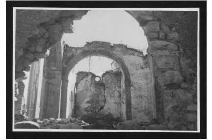
SC-016_13985_104.tif Damaged monuments P
