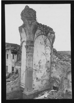
SC-016_13985_040.tif Damaged monuments P
