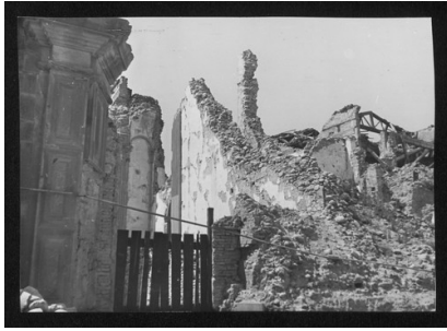
SC-016_13985_093.tif Damaged monuments P
