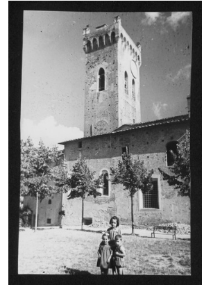
SC-016_13987_036.tif Damaged monuments S
