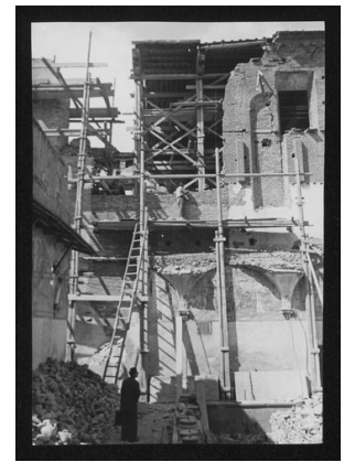
SC-016_13985_080.tif Damaged monuments P
