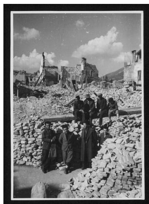
SC-016_13985_046.tif Damaged monuments P
