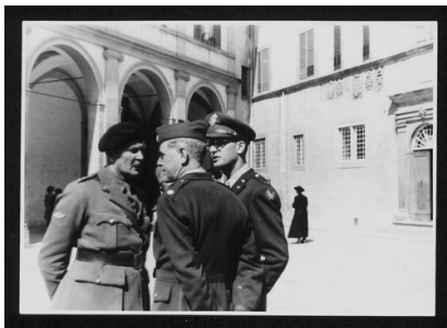
SC-016_13977_068.tif Damaged monuments C
