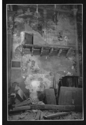
SC-016_13987_062.tif Damaged monuments S
