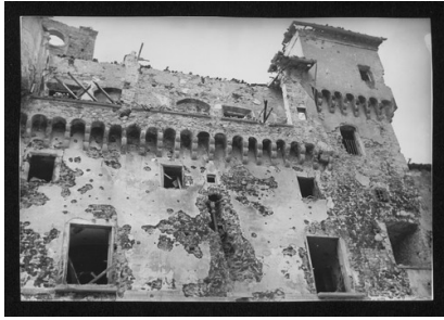
SC-016_13977_031.tif Damaged monuments C
