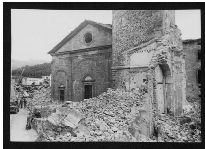
SC-016_13977_035.tif Damaged monuments C
