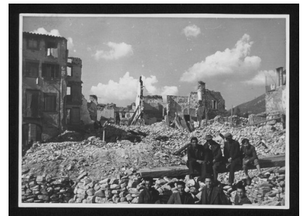
SC-016_13985_047.tif Damaged monuments P
