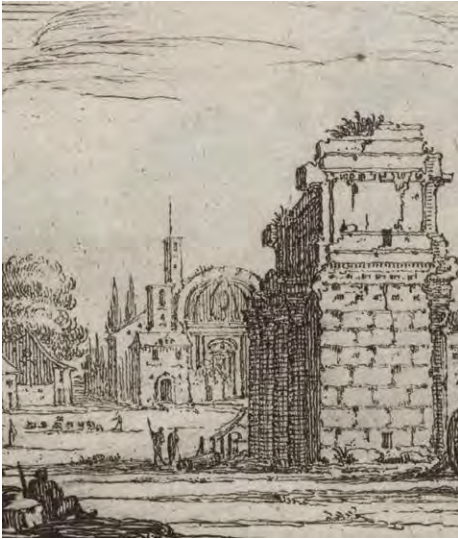
Israël Silvestre, View of the Campo Vaccino (1640–1660), detail of the Church of Santi Luca e Martina (under construction). National Gallery of Art, Washington, Gift of Robert H. Thayer
