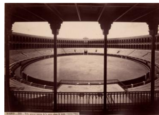
12 J. Laurent and Company, General interior view of the new bullring, Madrid, c. 1874
