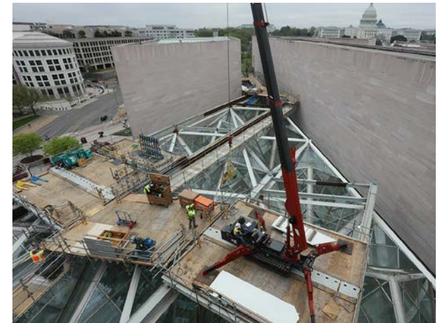
National Gallery contractors work to replace the East Building atrium skylights as part of the Master Facilities Plan.
