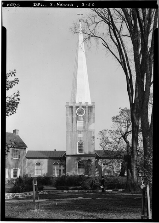
fig. 1 W. S. Stewart, West Facade—Immanuel Church (Episcopal), The Green, New Castle, New Castle County, DE , October 23, 1936, photograph, Library of Congress, Prints and Photographs Division, Washington, DC
